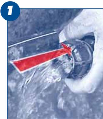
Assembly is so easy you can even do it under live conditions. Cut the pipe square and line up the pre-assembled fitting.
