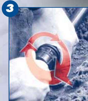
Tighten the nut with a turn of the hand and then firmly with a wrench.
