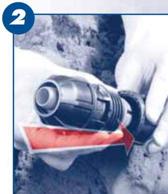
2 Assemble the fitting by pushing the fitting body over the insert and sliding the collet and the nut up to the insert shoulder.
