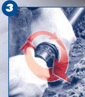
3 Position collet and nut, then turn to tighten. The fitting is fully installed when the nut can't be tightened further.
